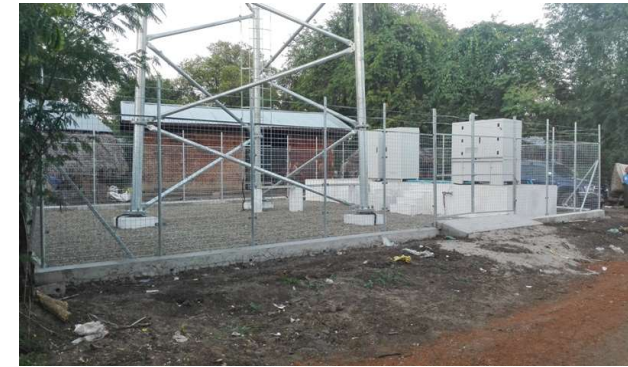
Ground Base Tower-Fencing Works
