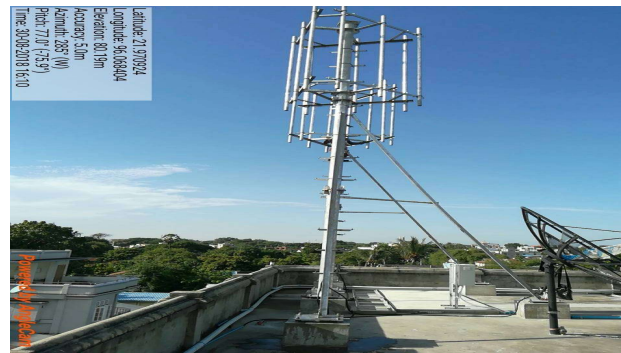
Roof Top Tower construction
