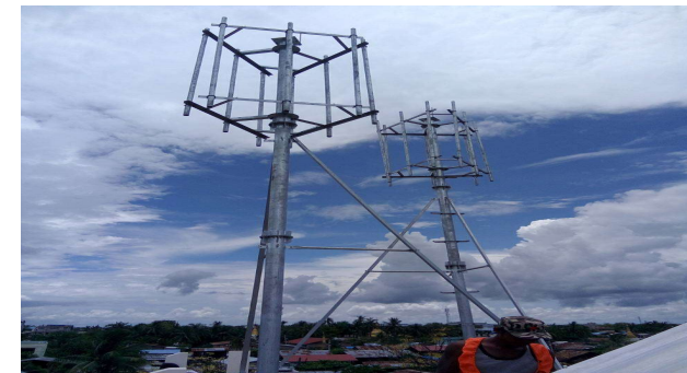
Roof Top Tower
